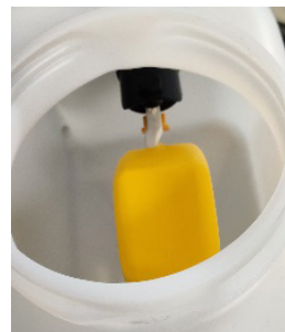
Picture 6.b Float valve in-side tank
